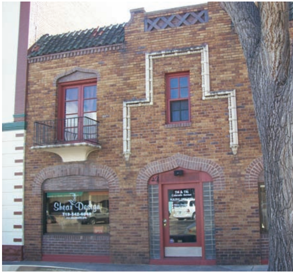
▲ Landmark. Jacob Gile designed this commercial property at 114 Colorado, which is not yet landmarked. Some property owners are ready to reap the benefits of landmarking, including tax breaks, access to grants, and increased property values. Still, landmarking is not the only means to preserve South Pueblo's architectural heritage. ( City of Pueblo )
