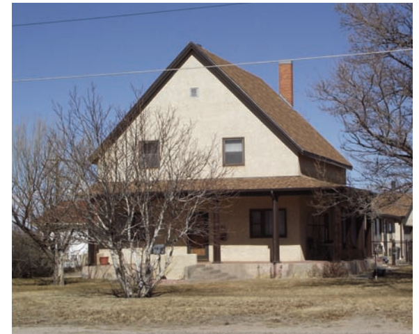
Figure 4.1. This house at 46 Carlile Place is likely the original William Moore house. (Jeffrey DeHerrera)
