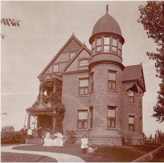
Figure 4.4 and 4.5. The Matthew J. Galligan home is a fine example of the Queen Anne style with its wrap around porch and circular tower. (Historic image courtesy of Anna Wade, contemporary image Jeffrey DeHerrera)
