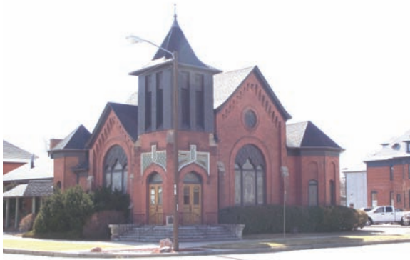
Figure 11.3. Prolific architect George Roe designed the First Methodist Episcopal Church. (Jeffrey DeHerrera)
