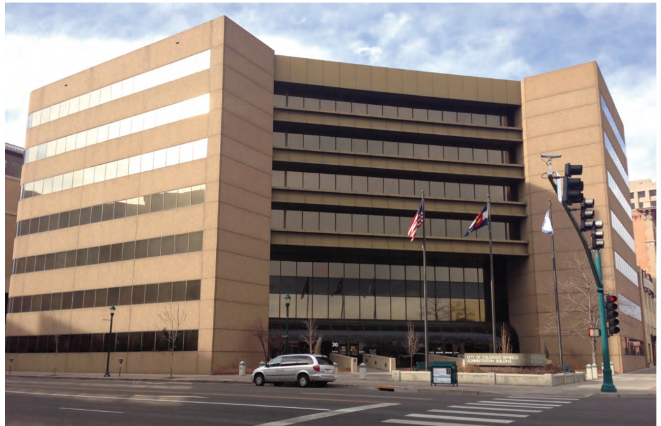
Figure c.1. The City of Colorado Springs Administration Center is indicative of the office buildings that have come to replace traditional city halls across the country. (Adam Thomas)
