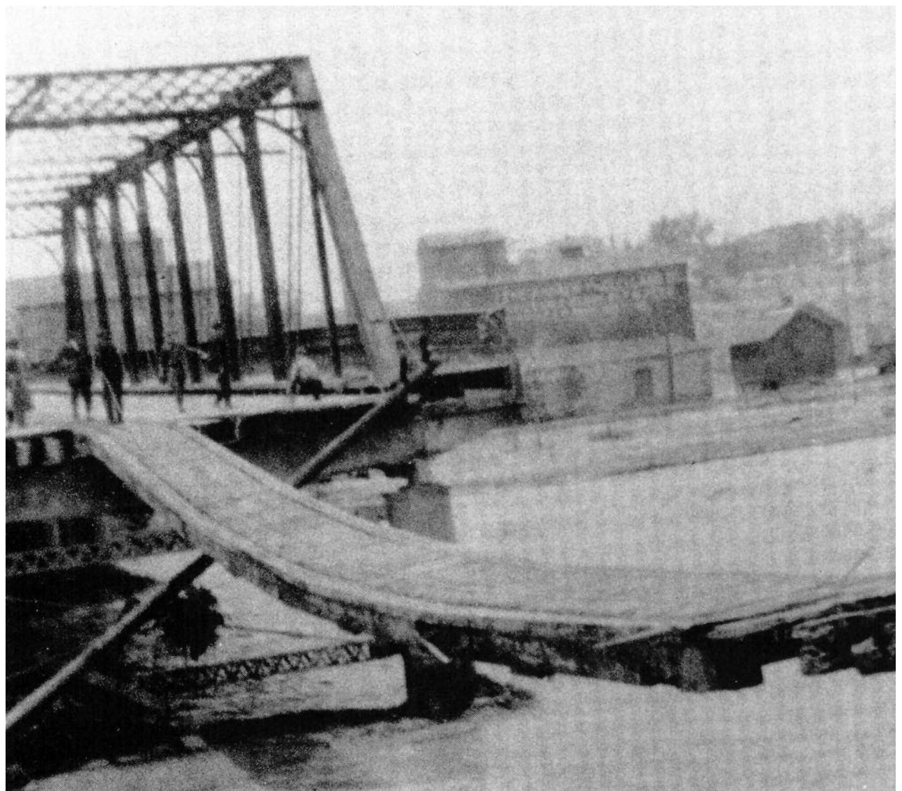
Figure 1.1. The 1921 flood wiped out the First and Eighth street bridges and the westernmost span of the Fourth Street bridge, leaving only the decking suspended between the streetcar rails. For weeks, this was the only means by which residents of East Pueblo could directly reach the rest of the city. ( Pueblo City-County Library District )
